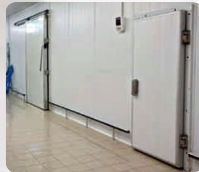
➤ Cold Room Doors
